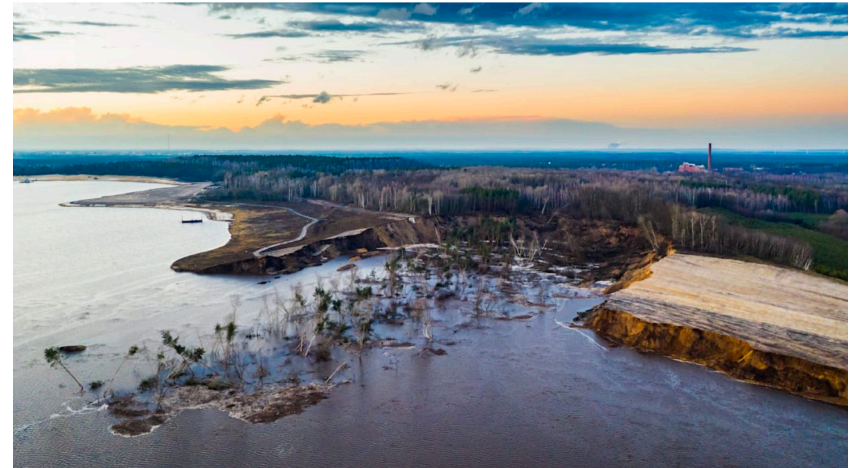
The aftermath of the landslide at Knappensee on 11 March 2021. Image by HY-photo Gernot Menzel via Bild .
