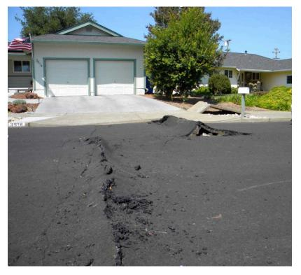
Fault damage in the suburbs west of Napa, California from the August 24th magnitude 6 earthquake. The fault rupture ran through homes and across roads, buckling the tarmac surface and pavements.
